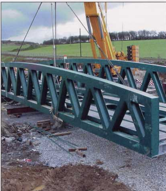
A complete hundred tonne bridge, profiled drilled and shot blasted and painted, supplied to an Irish client.
