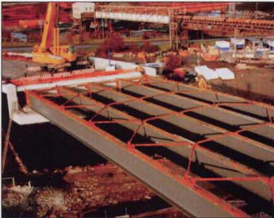
Typical plate girders awaiting erection for a steel framed building.
